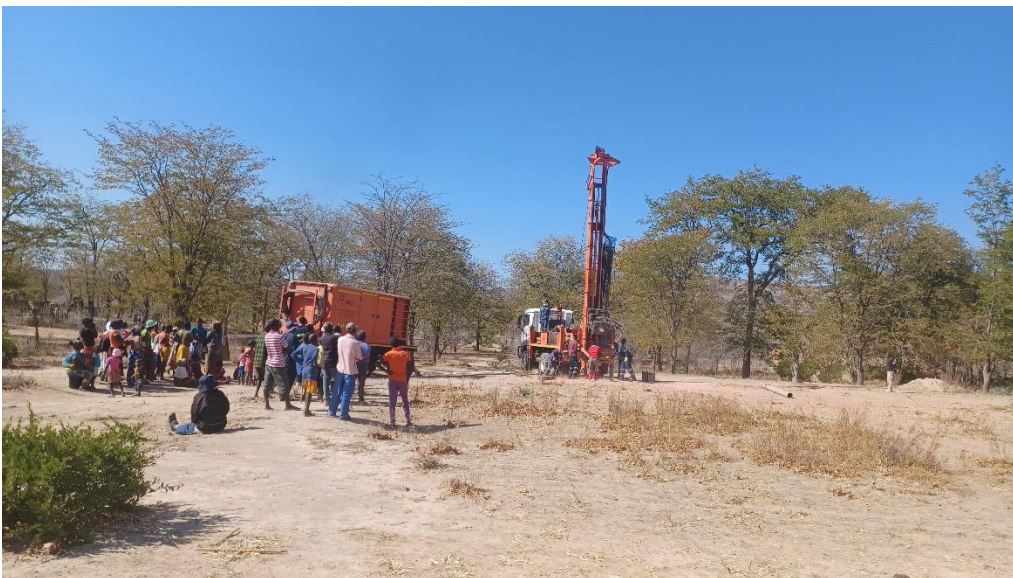
Drilling taking place with community members onlooking.
